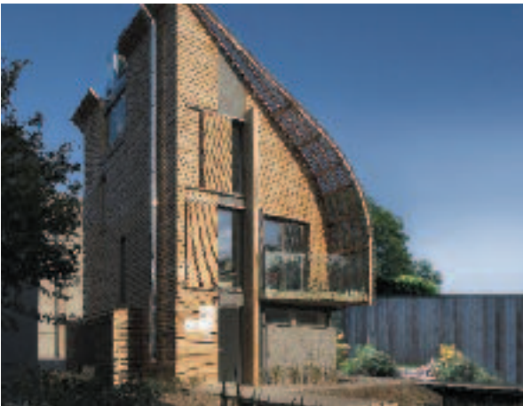
Kingspan Lighthouse, Watford
